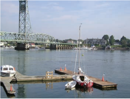
Strong currents sweep beneath Memorial Bridge - Prescott Park Dock, Portsmouth, NH
